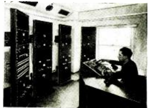
RADIO ROOM AT HOTEL LEXINGTON This set-up does not look much like the receiver in your home—does it!
